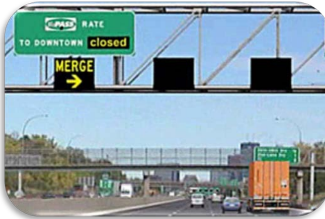
Figure 13. Graphic. Closing Priced Dynamic Shoulder Lane—Minneapolis, Minnesota. (27)
