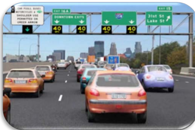
Figure 12. Graphic. Open Priced Dynamic Shoulder Lane—Minneapolis, Minnesota. (27)
